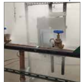
Water Ingress Testing
