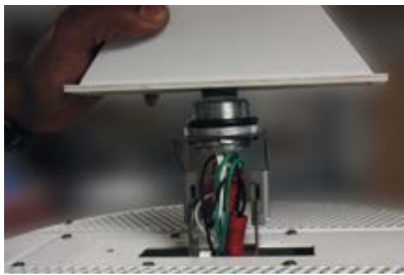
5. Make electrical connection, then slide cover down.
